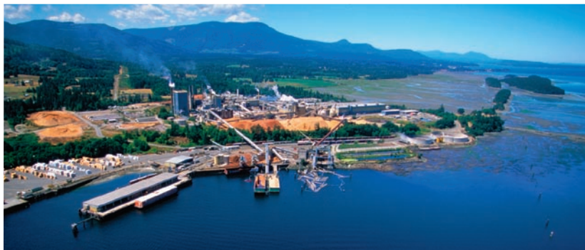
The Crofton mill on Vancouver Island has a long record of active energy and environmental management, and has made major strides in replacing fossil fuel with wood waste.
